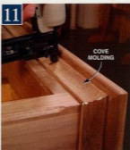
11 Attach the cove molding with pin nails or small brads. For additional strength, the molding is glued to the case and at the miters.
